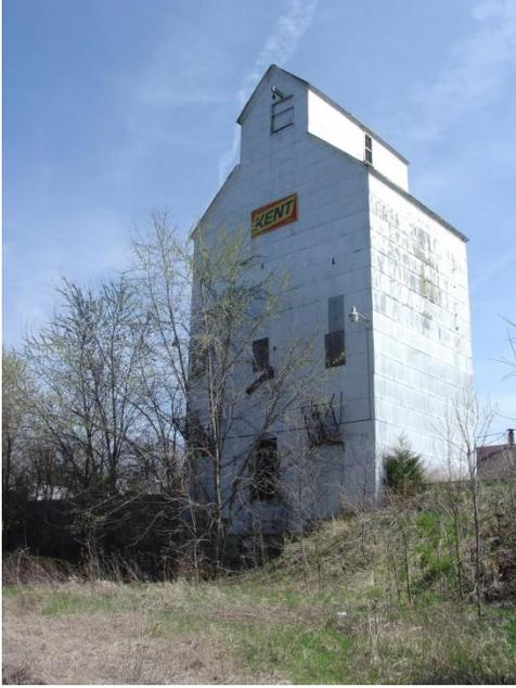
Grain Elevator dated circa 1870s or 1880s, is one of the last remaining wood stave built elevators along the railroad line. Debate remains as to whether to restore or demolish this historic structure.
