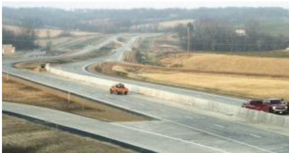
U.S. Highway 30 Bypass of Tama and Toledo
