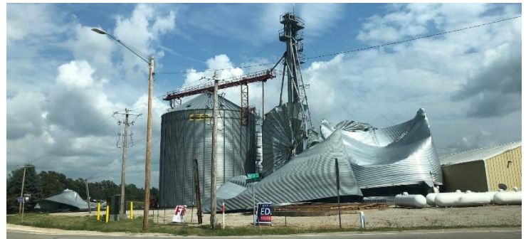
Marshall County grain bin damage from 2020 derecho. Source: Region 6 Resource Partners.
